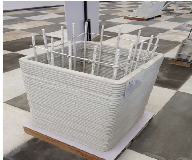
(b) The concrete mould printed
